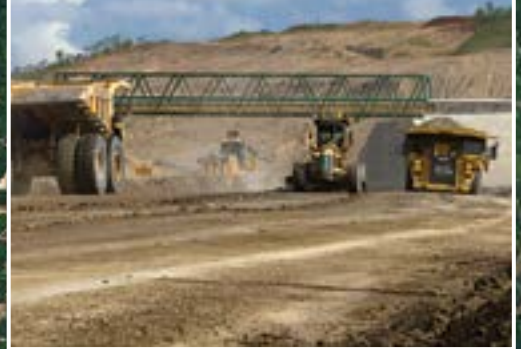
Indra Bridge, where the conveyor passes over a mine road.
